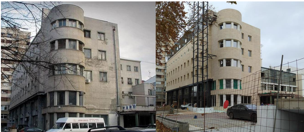
Fig. 5. Hotel Park in a state of decay (left) during the 2000s; Hotel Park in a process of redevelopment (right) in October 2020
